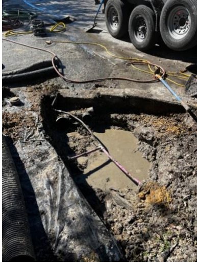
Photo 1 27 Jan 11:20 am - underdrain black pipes removed.
