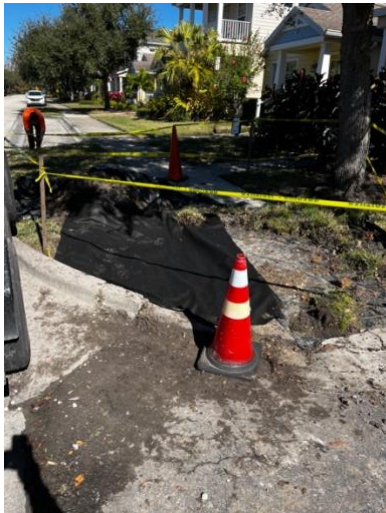
Photo 4 27 Jan 12:18 pm - top layer of new fabric added.jpeg
