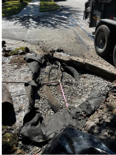
Photo 2 27 Jan 12:00 pm - new fabric under new black pipes installed
